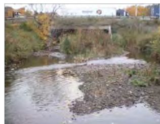
Existing twin cell culvert at Fletcher's Creek
